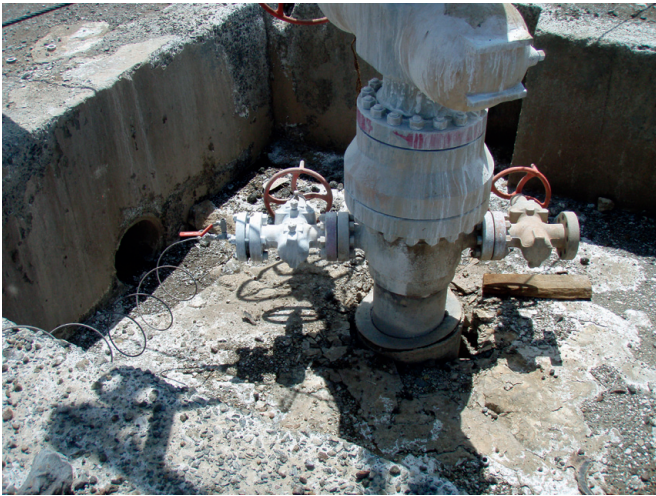
Fig. 4. Typical amorphous silica precipitates (white staining) at active high-enthalpy geothermal wells in the Rift Valley, Kenya, on 23 May 2012. (a) Silica scale on wellhead valve work and in the borehole cellar at Menengai No. 1 Production Well (capacity 8MW e ) of the Geothermal Development Company of Kenya (location: UTM zone 37M; Northings 9976800m; Eastings 171850m). (b) Silica scale on four steam–water separators, silencers and water removal pipelines serving the Olkaria No. 11 Production Well (capacity 9.6MW e ) of KenGen (location: UTM zone 37M; Northings 9900850m; Eastings 200240m).
