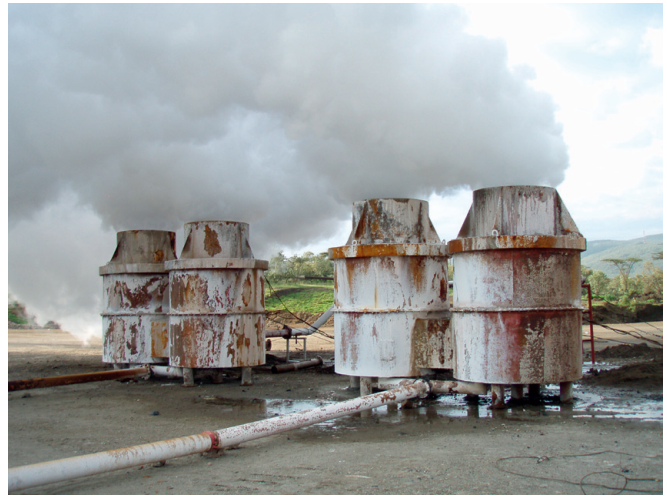
Fig. 4. Typical amorphous silica precipitates (white staining) at active high-enthalpy geothermal wells in the Rift Valley, Kenya, on 23 May 2012. (a) Silica scale on wellhead valve work and in the borehole cellar at Menengai No. 1 Production Well (capacity 8MW e ) of the Geothermal Development Company of Kenya (location: UTM zone 37M; Northings 9976800m; Eastings 171850m). (b) Silica scale on four steam–water separators, silencers and water removal pipelines serving the Olkaria No. 11 Production Well (capacity 9.6MW e ) of KenGen (location: UTM zone 37M; Northings 9900850m; Eastings 200240m).
