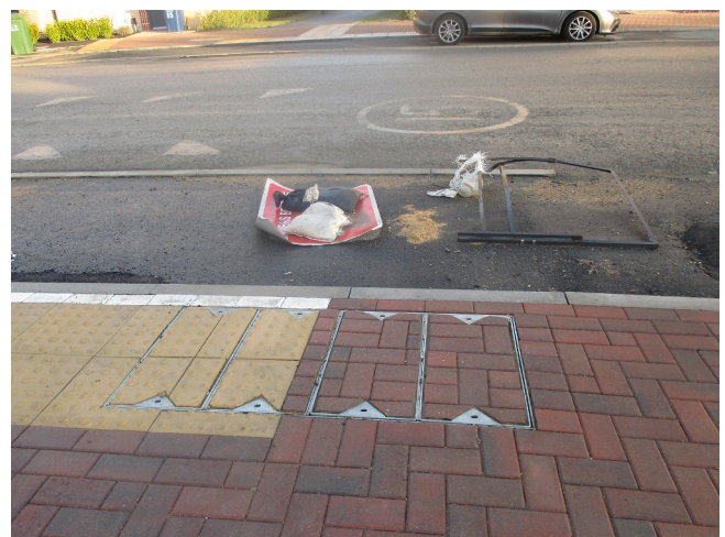
Fig. 2. Debris on the bike path “There is so much like this with the signs that have been blown over by the wind, or people have broken or just dumped them as you can see—that’s almost on the road. If that was to go on the road it would be very dangerous and it could easily be chucked on the road by the person who doesn’t care, and it just, that’s the cycle path thing again, and bikes will have to swerve around that.” (Bella, aged 12, Northstowe).
