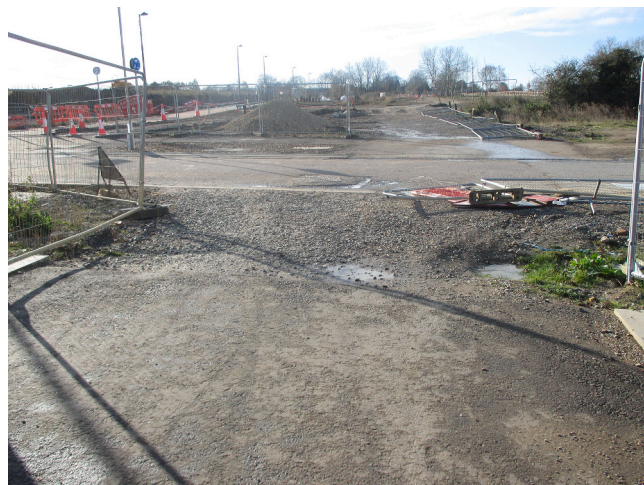
Fig. 7. Informal acts of care in the landscape of construction, photographed by Tom “ Yeah, this was where normally I stop and then I get on the like actual road to the school ... the helpful thing that I like is there’s builders there that tells the cars to stop so that’s good. ” (Tom, aged 12, Northstowe)
