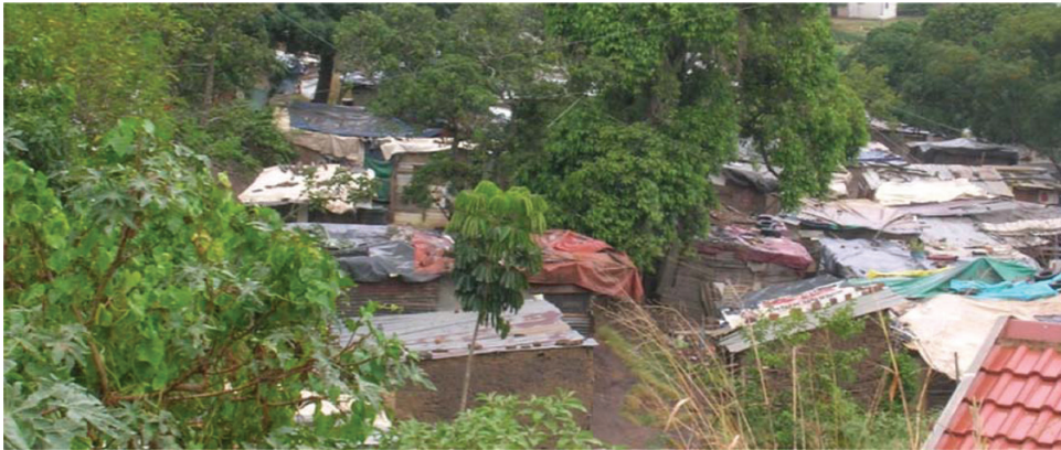
FIG. 4. The permeable roofs of informal houses.
