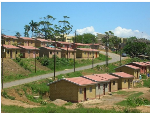
Figure 2. New RDP Housing in Cato Crest, Durban (Source: Meth, 2011).
