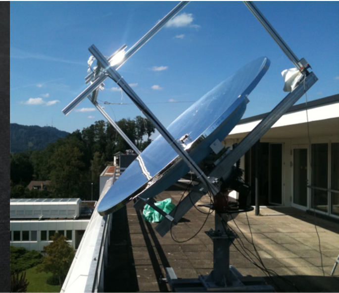
CPV System in Zurich
