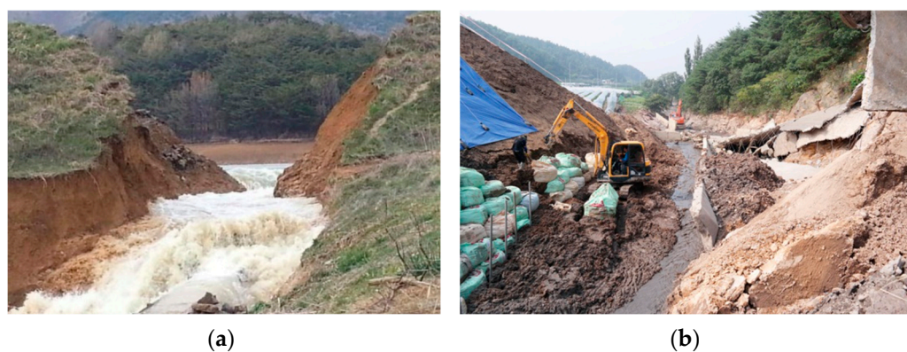
Figure 1. Dam collapses due to localized heavy rains in South Korea: (a) San-Dae reservoir; (b) Geo-Yeon reservoir.
