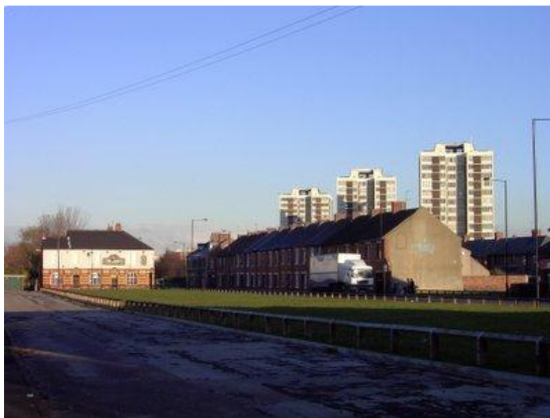
Figure 3 Houses and pub facing demolition, Walker Riverside, March 2006.
