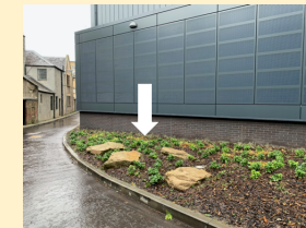
RAU exposure, in several pieces, beside a new building which was built after RAU was installed.
