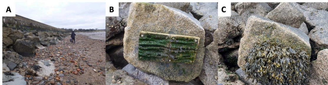
Fig. 2. A-C. Where A. Cross section view of the rock armour at low tide, MHWS is located just above the rock armour along the wall and MLWS is seaward of the low tide in this image (see Fig. 1); B. Colonisation of Ecotiles after 1st settlement seasons (March 2021) C. Colonisation of the same tiles after the second settlement season (September 2021).
