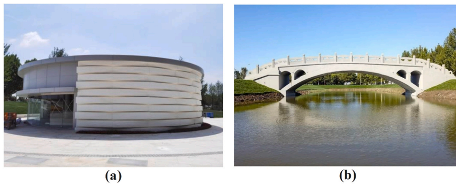
Fig. 18. Large-scale 3D printed structures, showing: (a) 3D-printed fabricated building in Nanjing and (b) 3D-printed concrete bridge in Hebei, China (reproduced from Refs. [235,245]).
