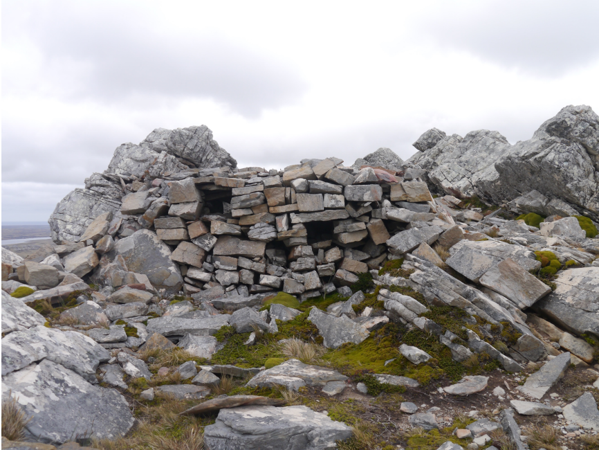
FIGURE 3 Drystone bunker built from angular rocks on Tumbledown – the closest that the author has seen to a pillbox on the islands PHOTO: TONY POLLARD
