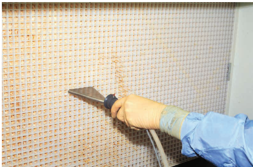
Figure D1: A probe scanning over a filter face to locate a leak
