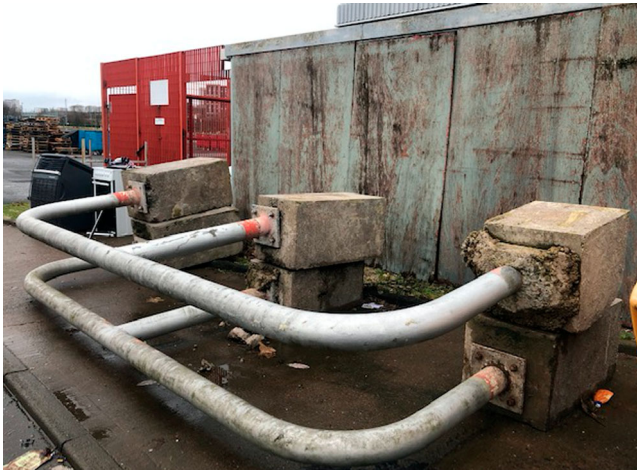
Figure 5. Upturned concrete barrier after COP26. (Source: Author's own photograph.)
