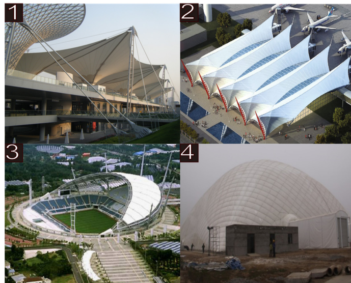
Figure 3. The main types of membrane structures: 1. Tensioned membrane structure, 2. Cable-membrane structure, 3. Skeleton membrane structure, 4. Inflatable membrane structure [12,30–32].
