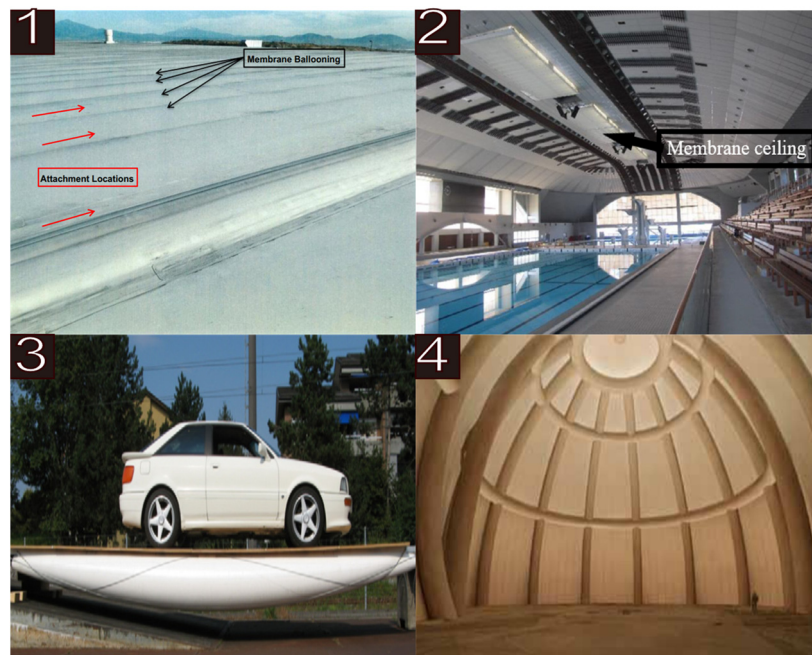
Figure 4. Other types of membrane structures: 1. Membrane roof, 2. Membrane ceiling, 3. Tensairity, 4. A movable laboratory [5,7,34,36].
