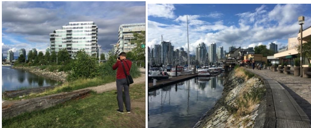
Figure 11: Alternative softer promenade (compared with hard edge) from Vancouver, Canada where the Left image (c. early 2000s development) has a much more organic and adaptable (as sea level rises) land-sea boundary with space to move the path landwards compared to the Right (c. 1980s) where saltmarsh plants in the hard engineered seawall appear as weeds and there is little or no accommodation space on land.
