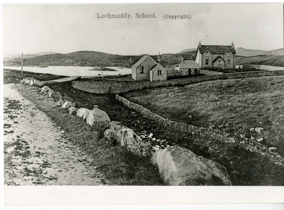
Fig. 2. Lochmaddy School, North Uist, built 1879, photographed in 1897. Copyright: Leabharlann nan Eilean Siar.
