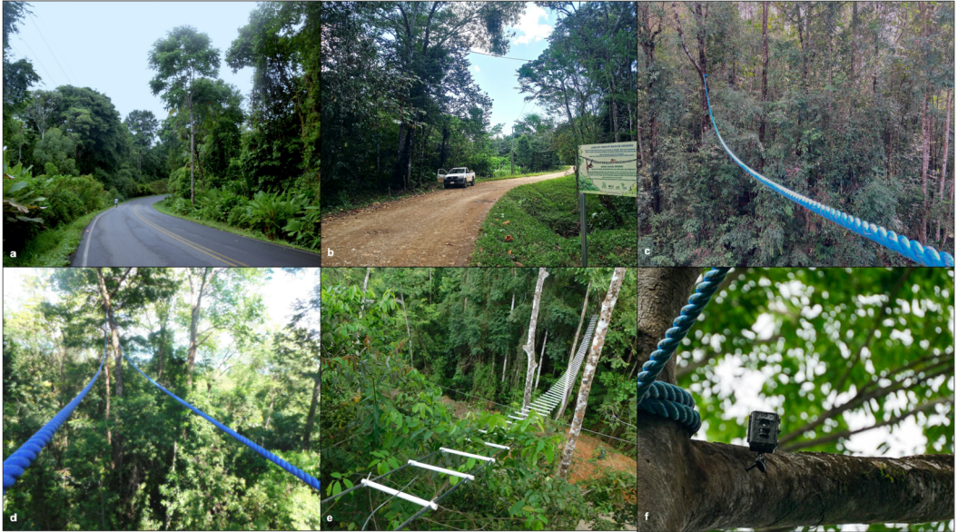
Figure 2. Osa’s road types, bridge designs installed and monitoring approaches: (a) Paved highway, (b) Gravel/dirt road including citizen science monitoring sign, (c) Single rope bridge, (d) Double rope bridge, (e) Ladder bridge, (f) Camera trap monitoring of bridges.
