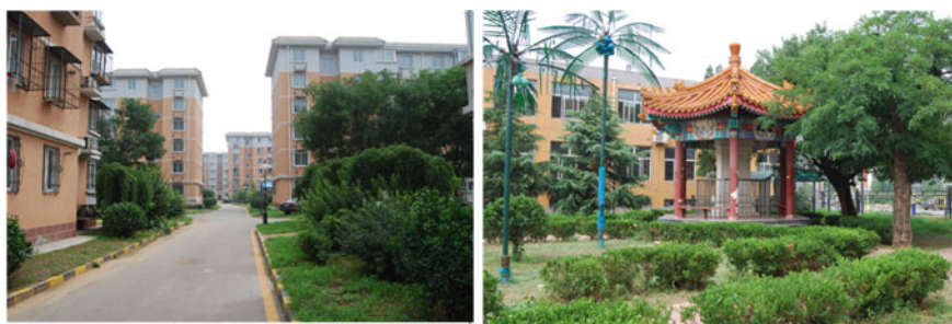
Fig. 6.4 Replacement flats in WSY (left) and new Village Committee office (right)
