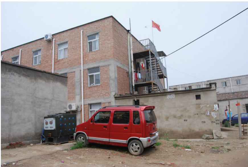
Fig. 6.2 A new house built inside the half-demolished village
