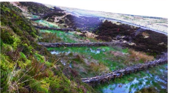
824 Figure 2: A) Two Lads Study Site Photographs Prior to WELJ installation; B) the site follow- 825 ing WELJ installation
