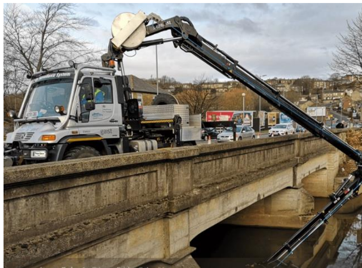
Figure 23. Bridgecat technology for bridge inspection [89].
