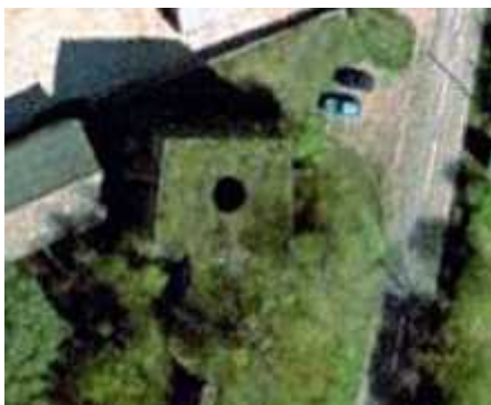
Figure 13. Google Earth image of the draw line at the Cults Lime Works (eastern Scotland). Note the massive square masonry structure surrounding and supporting the line (the central circular feature).
