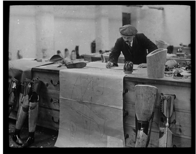
Figure 3. Designing artificial limbs. Engineers from the Clydeside shipyards were integral in the design process. University of Glasgow Archives reference DC079/173.
