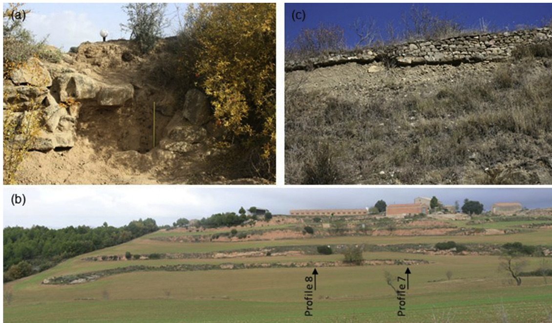
Fig. 2. Representative photos of the terraces and sediment stratigraphies examined: (a) the Balaguer check dam (see Fig. 4); (b) the braided terrace network at Els Prats de Rei; (c) a stepped terrace at the Castell de Mur.
