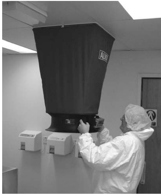
Figure 1 Airflow measuring hood used on a diffuser in a cleanroom
