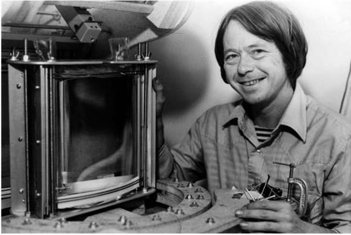
FIG. 4 Alternative technologies: Lloyd Cross, circa 1975, with cylindrical lens fabricated from Plexiglas and mineral oil. (Museum of Holography Collection, MIT Museum.)
