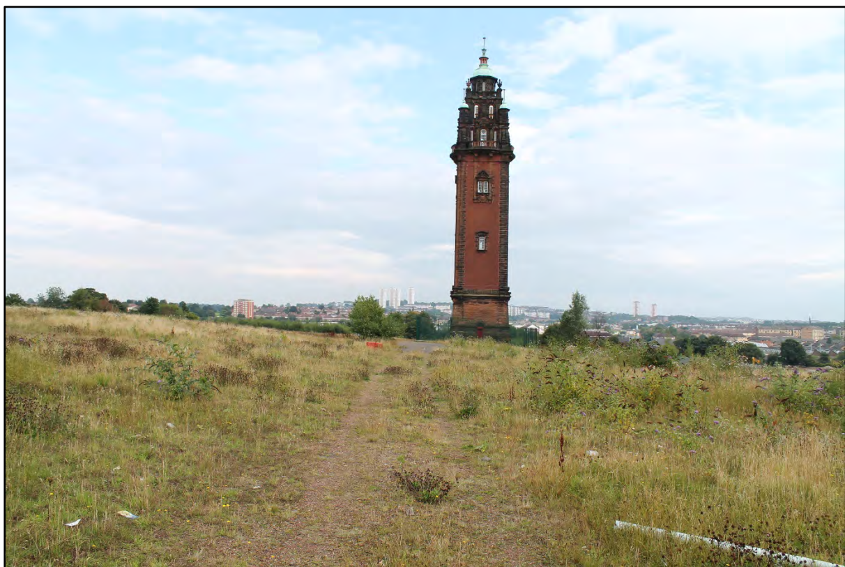
Figure 2: Derelict land at the former Ruchill Hospital, North Glasgow
